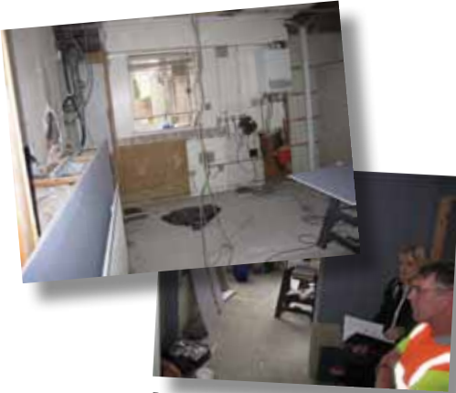
Refurbishment of Balcarres Street in progress
